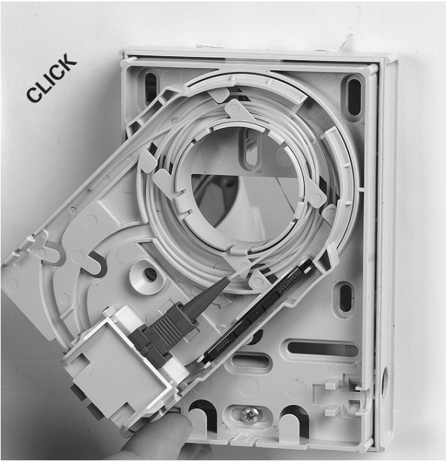
1.2.11 Rotate until the tray is touching the faceplate. Still keeping the fibers under low tension when installing the tray onto the face plate, so that fibers will stay inside the storage area during the installation.
