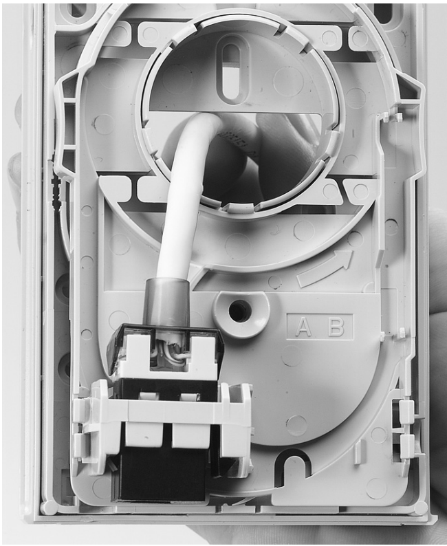
1.2.16 Termination of a CAT cable.
