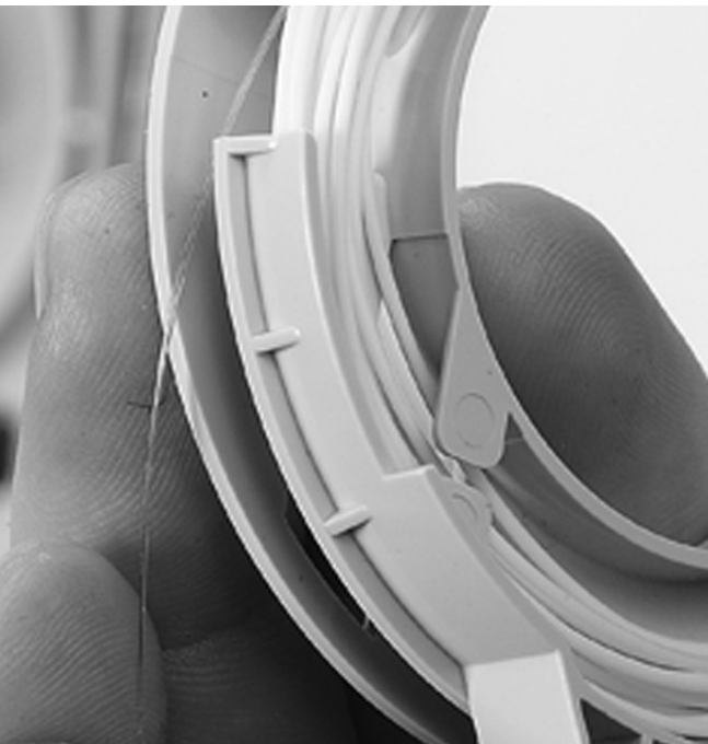
1.2.9 Route the feeder cable fibers to the backside of the tray as shown in the pictures.
