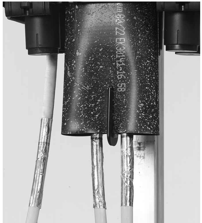
5.1.4 Push the sleeve against the base and place the clip.
