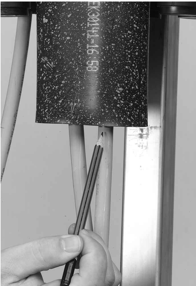
5.1.2 Remove the packing bag out of the sleeve, push the sleeve upwards to the base and mark the cable flush with the sleeve. Make sure the non-coated zone butts up against the base.
