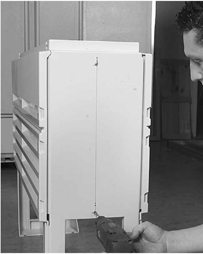
9.1.7 Drill the two holes (Ø 8.5 mm).
