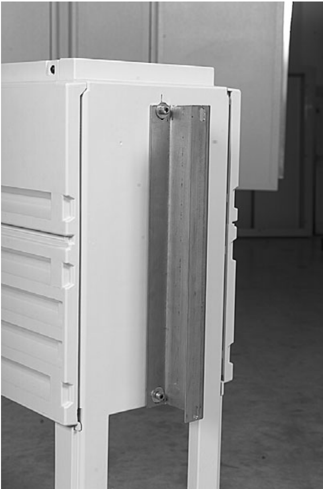
9.1.8 Install the connection kit and tighten the nuts (20-25 Nm).
