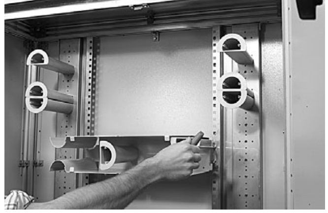
4.2.2 Mount the POM (Pigtail Orientation Module) at the correct location (depending on the configuration).
