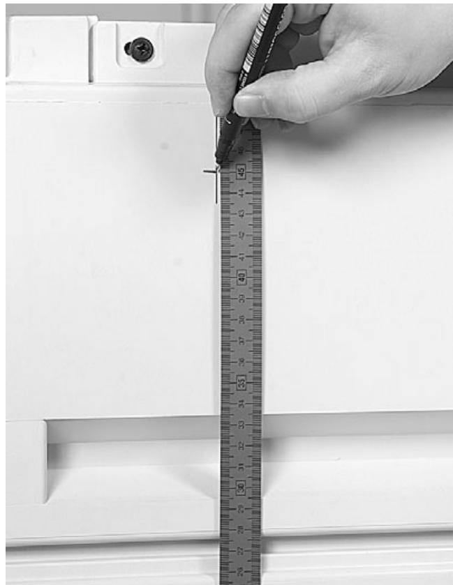
10.1.4 Start at the bottom, first mark at 15 mm, second at 450 mm.
