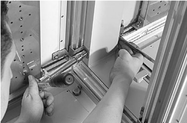
9.2.8 Fix the two cabinets with the connection frame in between. Tighten the screws between cabinet and pedestal (20-25 Nm).
