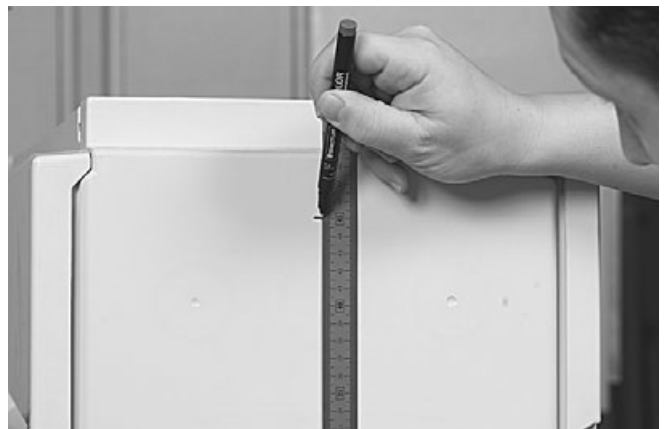
9.1.6 Start at the bottom, first mark at 15 mm, second at 450 mm.
