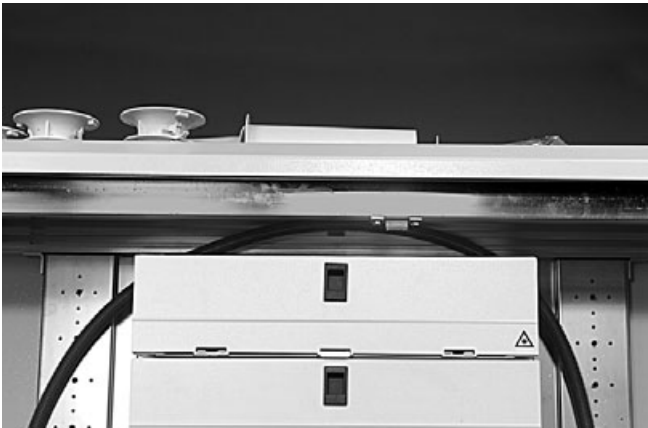
5.3.4 In case of cables coming from the left: route the flexible tubes under the bottom shelf (preferably) or over the top shelf.
