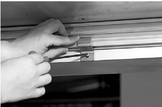
10.2.6 Fix the connection frame temporary with the bracket.
