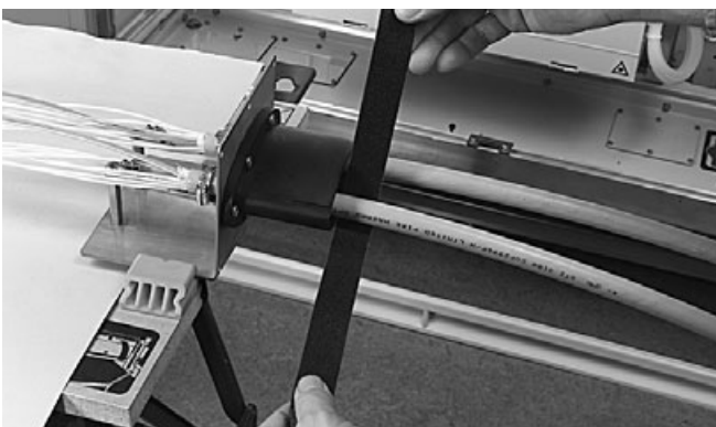
5.4.8 Abrade the oval port and the cable over a distance of 150mm from the end of the port.
