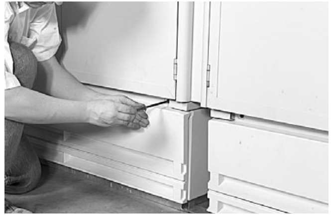
9.2.9 Place the cover on the pedestal.
