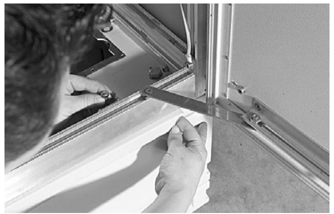
9.2.10 Place the protection plate back.
