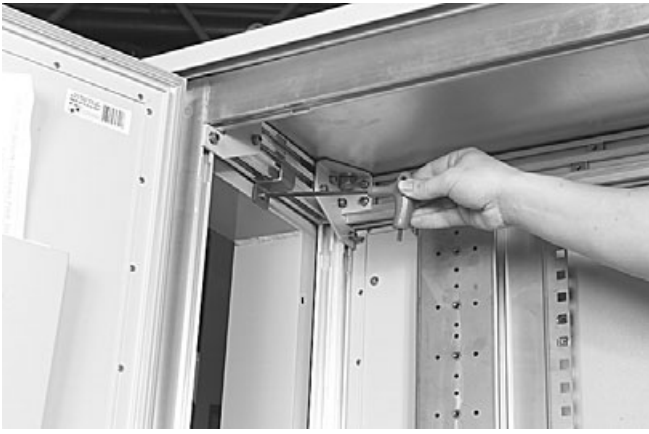
9.2.6 Fix the connection frame temporary with the bracket.
