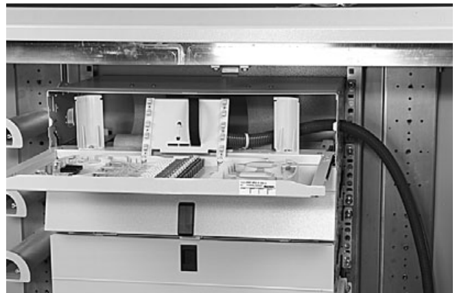
5.3.3 In case of feeding a cable to a GPS2: guide the flex straight to the shelf, allow some slack for sliding the tray.
