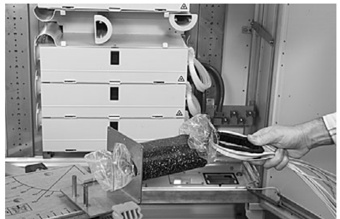
5.4.4 Take the looped cable installation tool (LCIT, to avoid kinking of the loose tubes) and place it in the middle of the window cut. Bend the loose tubes around the tool and slide it inside the heat shrink tube and the oval port. Protect the inside with the PE bag to avoid dirt and grease coming in contact with the hot melt inside the sleeve. The printed arrow on the sleeve should point towards the outlet flange!
