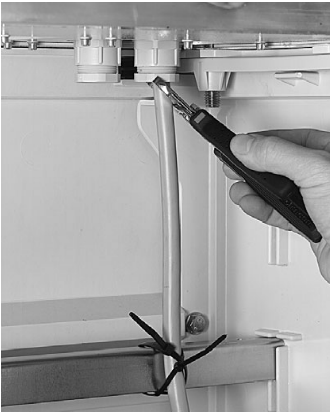
5.2.4 Fasten the seal and fix the cable on the metal bar using 2 tie-wraps.
