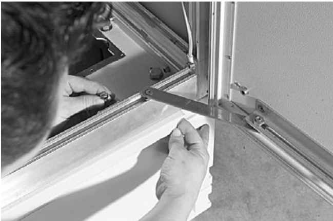
10.2.10 Place the protection plate back.
