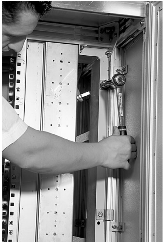
10.2.8 Fix the two cabinets with the connection frame in between. Tighten the screws between cabinet and pedestal (20-25 Nm).
