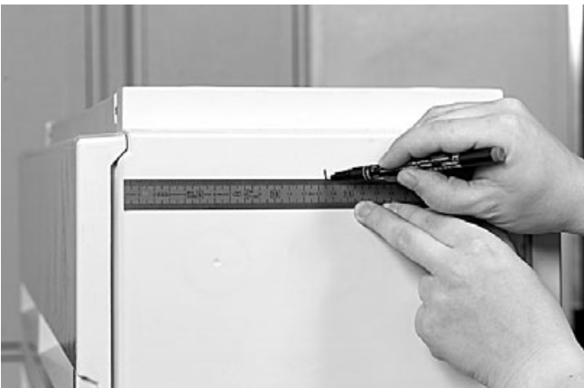
9.1.4 Mark the side of the pedestal in the middle.
