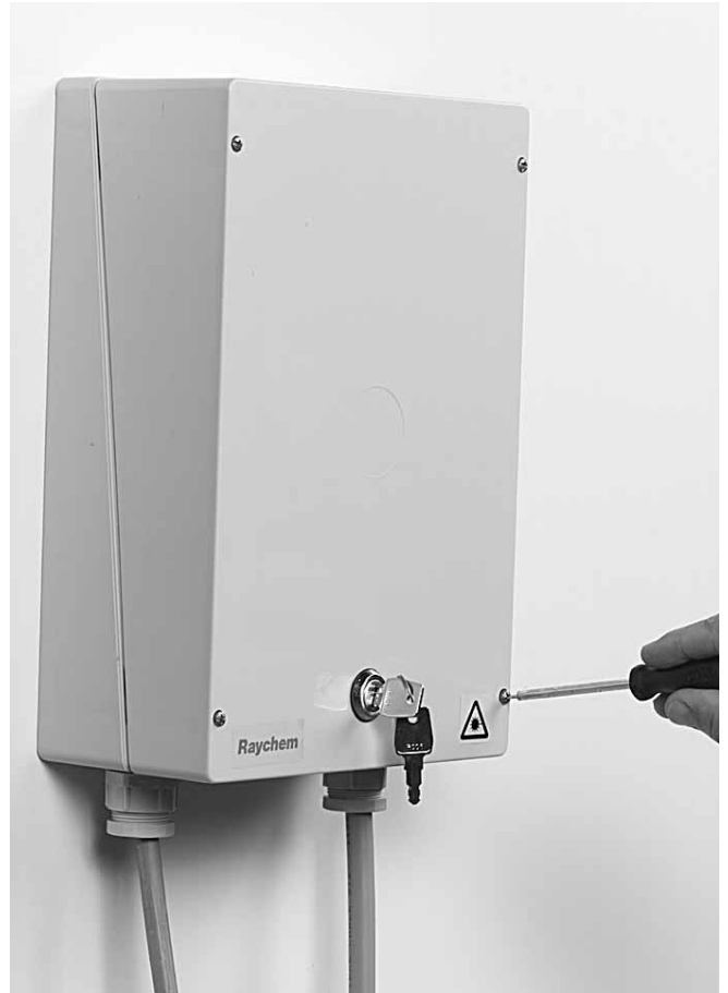
7.3 Place on the cover on the box base and secure the cover with the screws.
