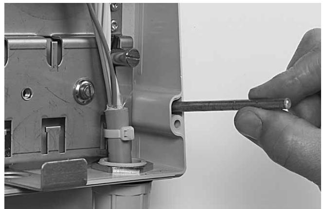
7.4 In case of a box with lock insert first the four guiding pins in the box before installing the cover.
