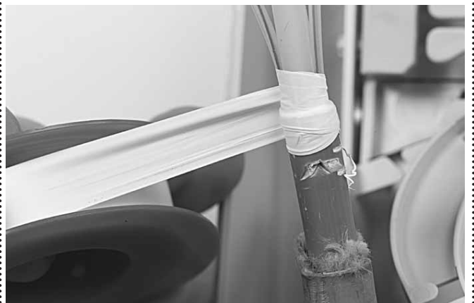
4.1.3.2 Protect the transition from the cable to the tubes with a few layers of Teflon tape.
