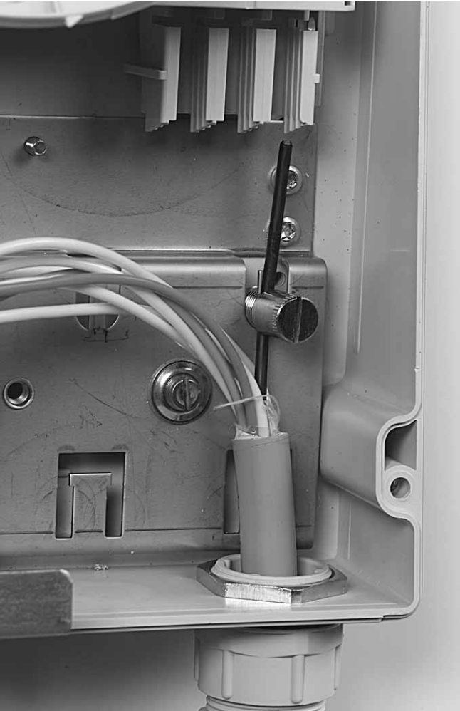
4.2.1. Pull the cable back in the correct position, the cable jacket should protrude 30 mm into the box passing the cable strapping point.
