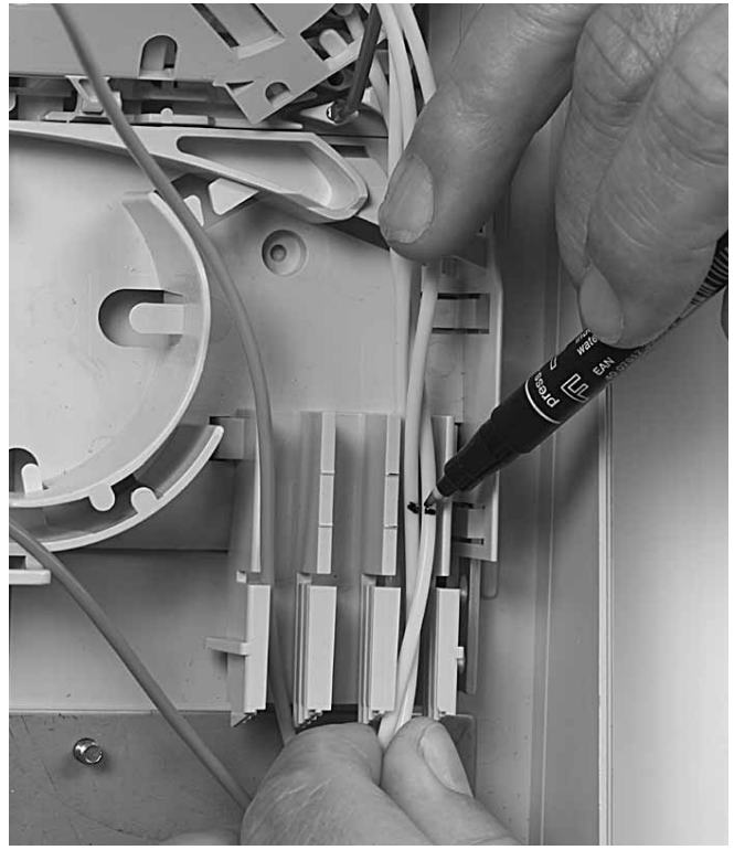
5.2.2 Mark the tubes between the two marks on the tubeholder.
