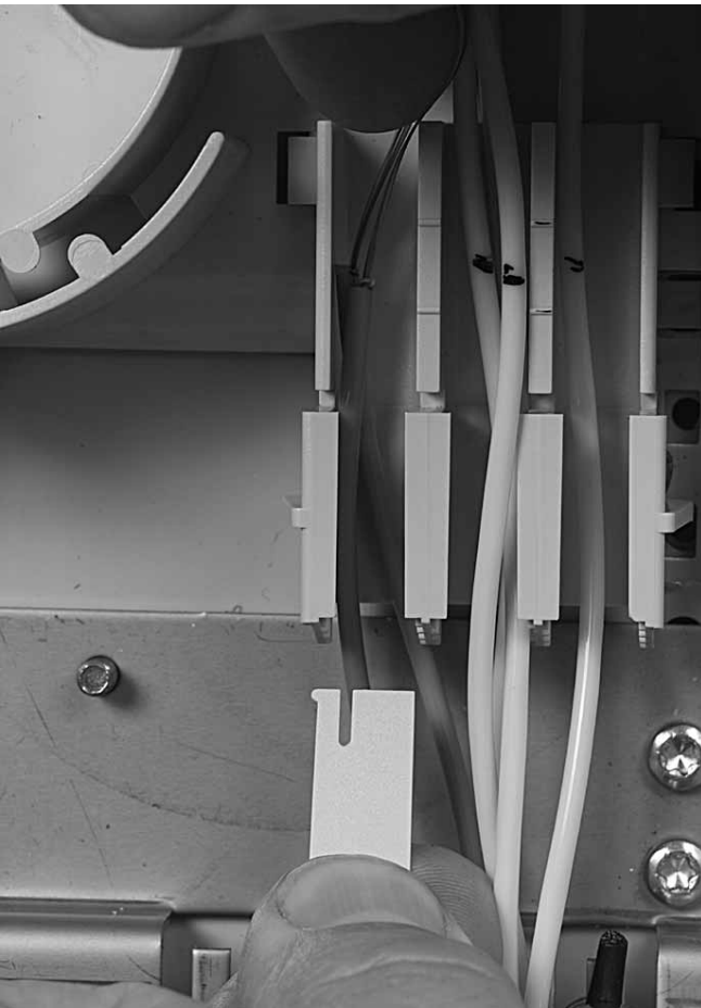
5.2.4 Position the loose tubes in the tubeholder and slide the tube holder retainer with the snap forwards in the lowest possible cavity of the tube holder above the loose tubes. The tube holder retainer must snap.
