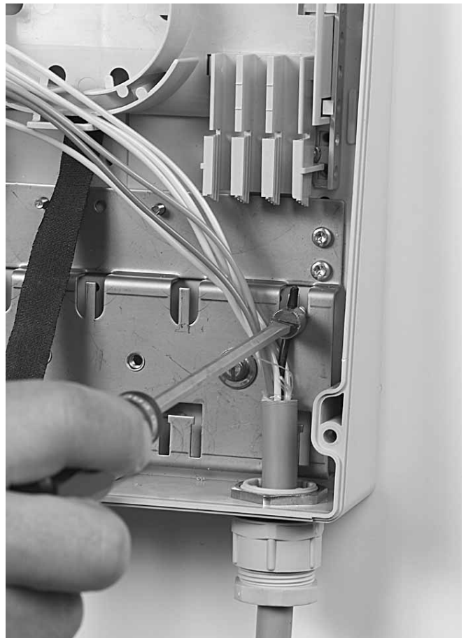
4.2.2. Insert the strength member in the strength member connector and tighten the connector with a screwdriver. If necessary, remove the plastic core from the strength member till it fits in the strain relief connector.
