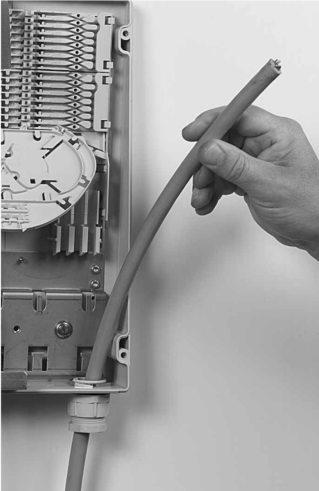
4.1.1. Feed the cable through the cable port gland.
