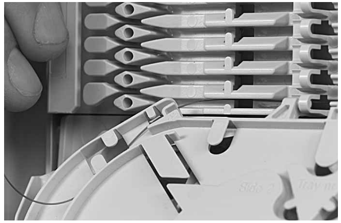
5.2.6 Pull gently on the fibers in the tray and make sure that the fibers are well contained in FAS block and wraparound groove plate.
