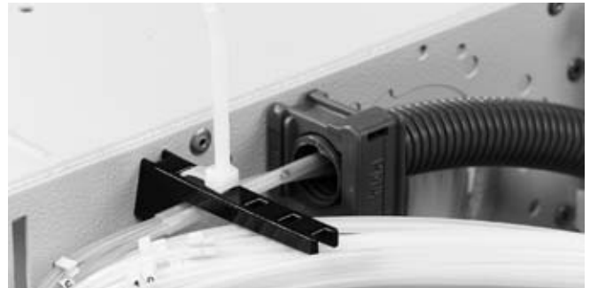
4.1.16 If no more loose tubes have to be terminated, cut the unused tubes. Secure the tubes with a tie wrap.
