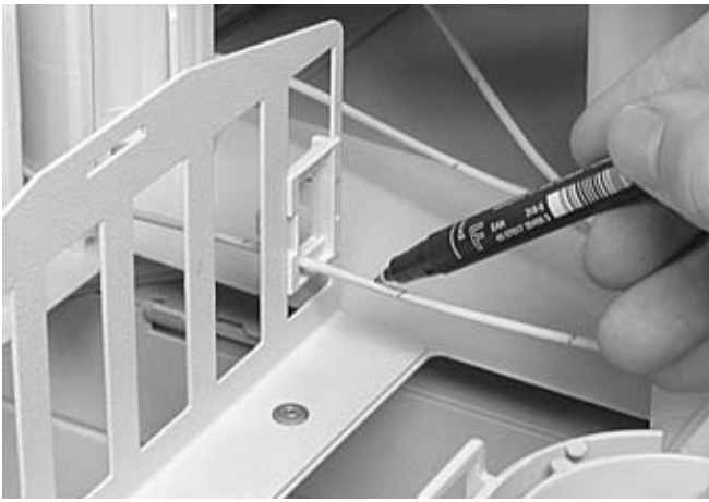
5.2.3 Mark at 5 cm from the bracket to have some slack for sliding the tray.
