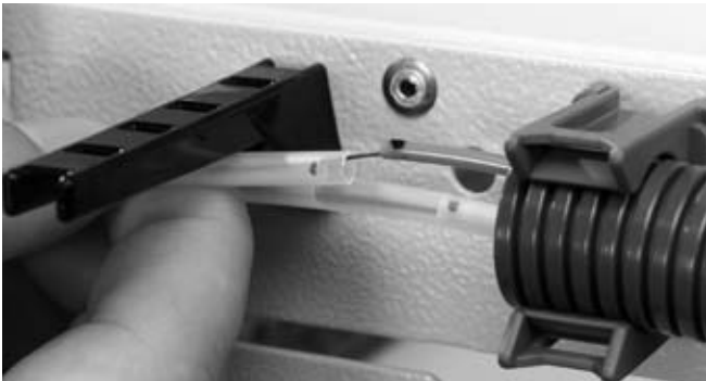
4.1.13 Select the loose tube and slide a 75 mm long FOPT-CT over the transportation and loose tube or the transportation tube directly over the loose tube.
