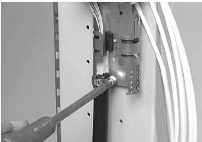
4.1.24 Secure with the cable clamp. Don't squeeze the cable.
