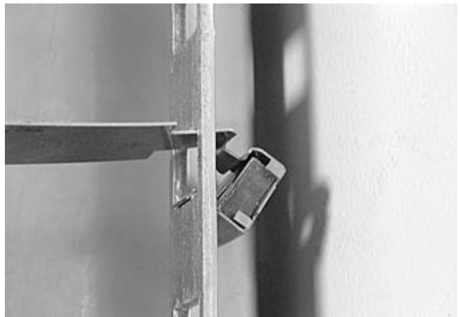
3.1.2 Determine the position of the unit (see rack installation instruction) Fix the cage nuts into the rack mounting uprights.
