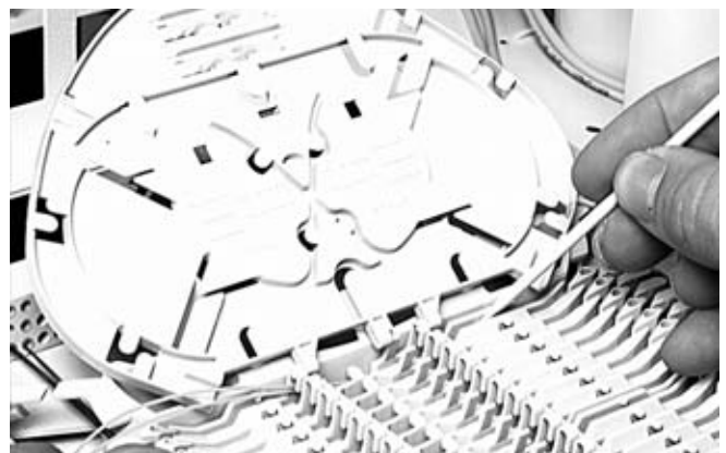
5.3.1 Guide the fibers into the corresponding groove. Make sure all fibers are positioned under the lips.
