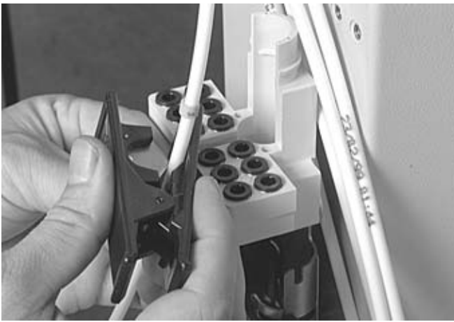
4.1.28 Cut the tubes to length using the tube cutter. Make sure the shelf is in an opened position.
