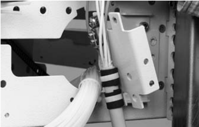
4.2.3 Strip the cable over 3,5 m. Cut the strength member at 35 mm from the outer jacket. Apply foam tape at the tie wrap positions. Install the prepared cable on the side termination plate.
