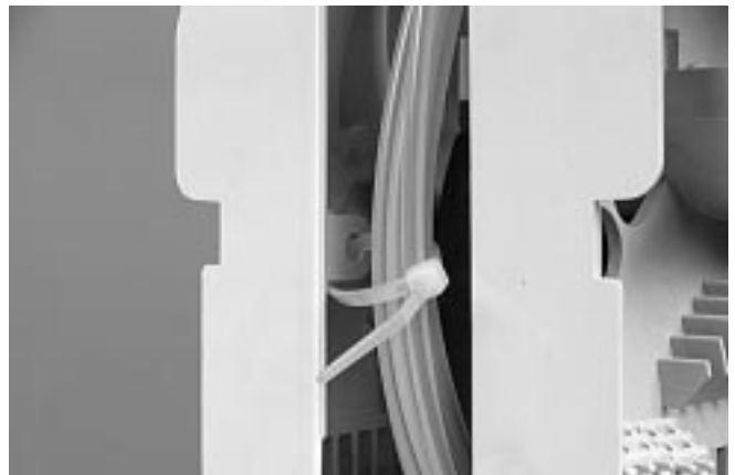
11.18 Bring together the FOPT-CS protection tubes with tie wraps on the FAS plate eyelet.
