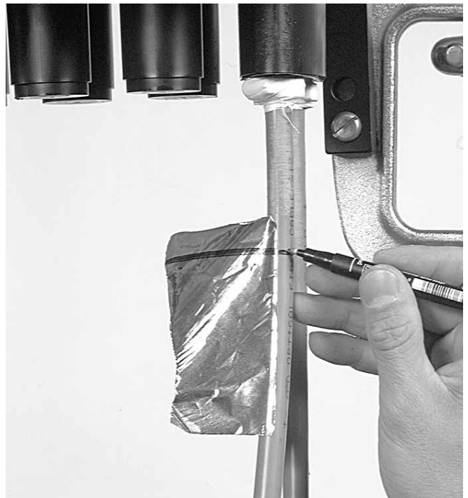
5.1.4 Match the blue line of the aluminium protection foil with the marks on the cables. Wrap aluminium cable protection foil around the cable (the aluminium foil should not be more than 30 mm inside the sleeve).
