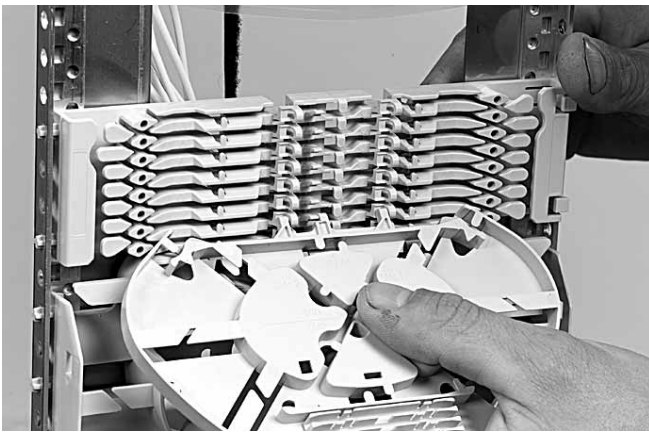
6.3 To remove push the two snapfits at S2 UMS-profile and slide the wraparound plate towards S1 UMS-profile.
