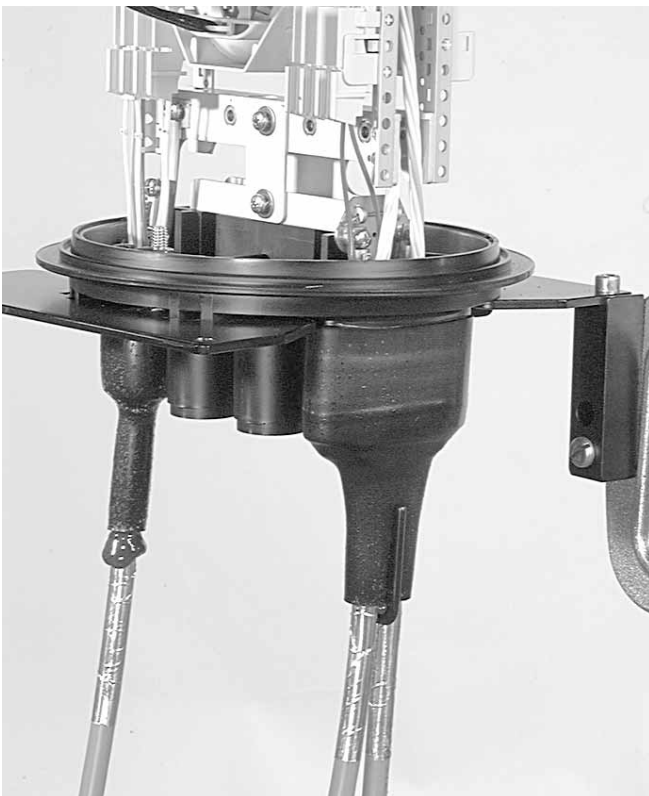
5.1.7 Hold the cable in position. Shrink till the green painting dots become black, and the hotmelt is visible on the end of the sleeve. Postheat the clip on both sides till the adhesive shows a proper flow on the clip between the two cables.
