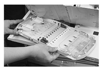
2.2 Secure the splitter tray into the sub-rack by pushing it into the hinge. Make sure the tray is inserted in the correct way (numbers 1-12) readable from the front.
