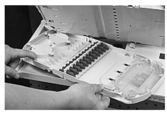
2.1 When necessary, one can remove the appropriate tray by pulling it out of the hinge.
