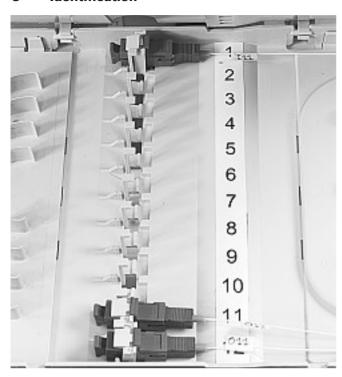
3.1 Connectors are numbered from 1 till 12 as shown on the picture.
