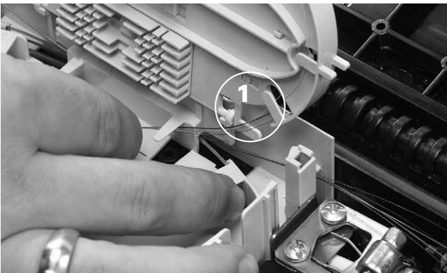
5.18 Route the fiber from the SMOUV holder to the storage area over the edge of the cassette leaving no slack through the opening (1).
