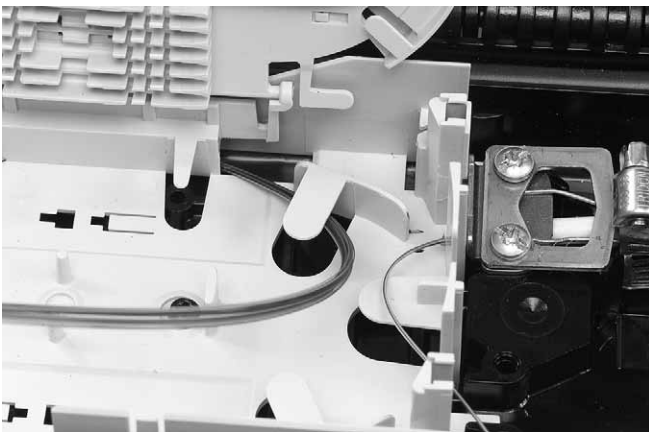
5.8 Route the incoming fiber into the groove behind the hinge of the tray to the storage area.
