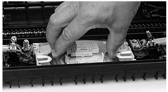
5.7 Install the splicing tray cover.
