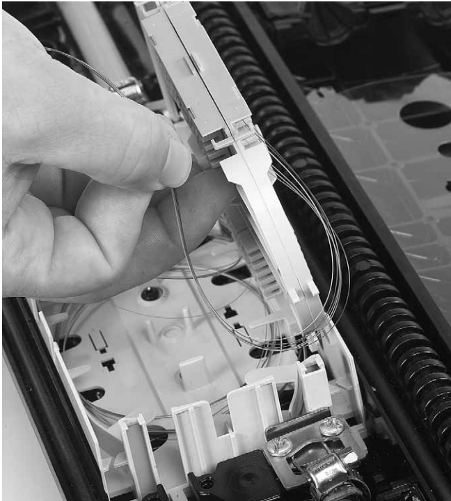
5.19 Place the fibers underneath the lips.
