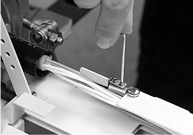
7.2.4 Slide sealing tube (included in kit) over cable, push strengthmember in strengthmember attachment and tighten screws.
