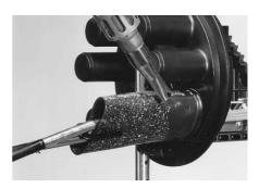
6.7 Shrink down the end of the sleeve on the cable side. Heat until the sleeve shrinks down on the cables and take care that the green thermo-indicating paint is converted to black. Postheat the clip on both sides till the adhesive shows a proper flow on the clip between the two cables.
